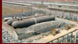
Diagram of Mounded Storage Vessel
